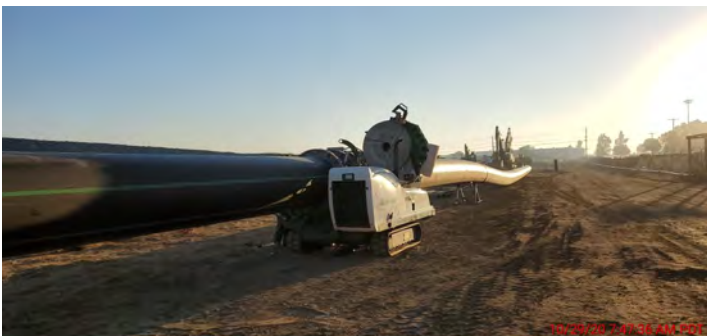
Fusing Reach IV-B By-pass Pipe
