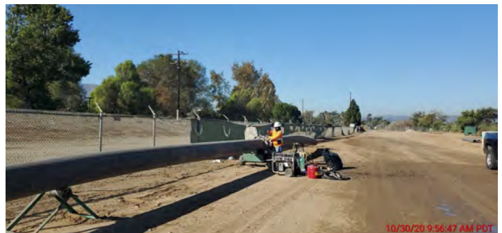
Fusing Reach IV-B 36-inch HDPE Pipe
