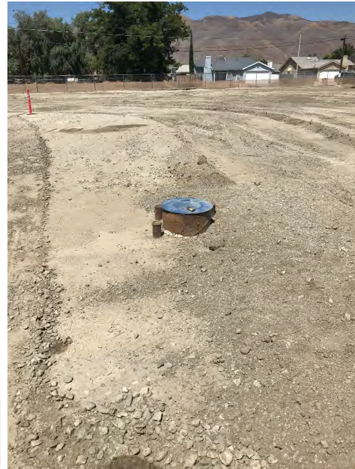
Well 201 - Photo Shows Well Head, Equipping Phase Next
