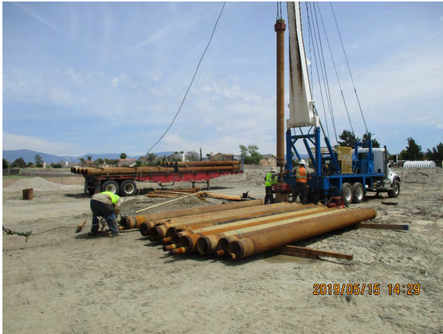
Well 201 - Drilling Complete, Photo Shows Test Pump Being Installed
