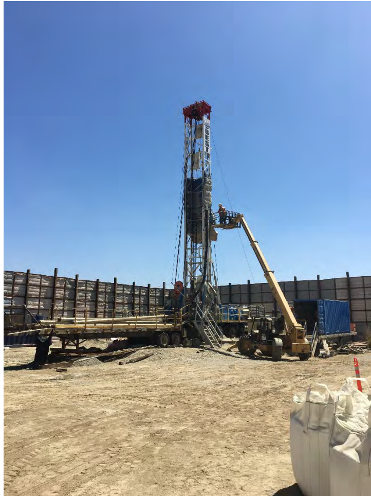
Well 203 - Photo Shows Well Reaming
