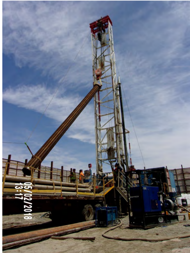
Well 202 - Drilling Complete, Photo Shows Casing Being Installed
