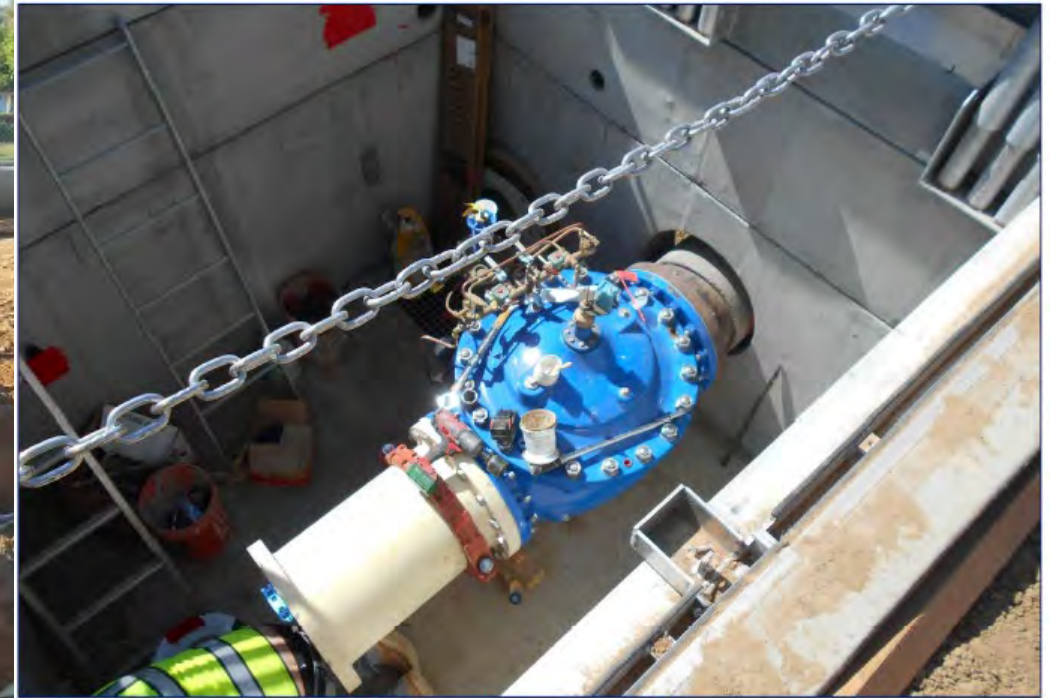
Valve Installed in Flow Control Vault
