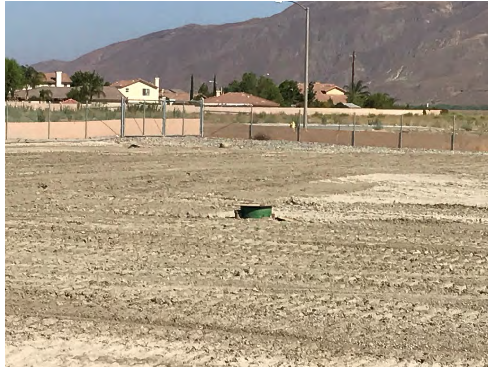
Well 202 - Grading Complete, Photo Shows Well Head, Equipping Phase Next
