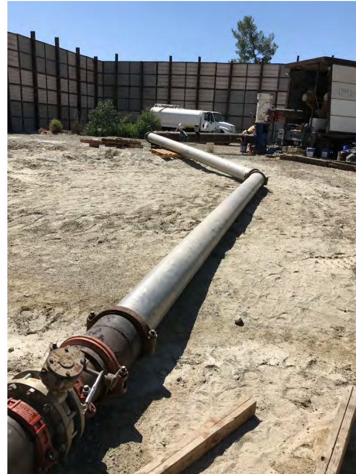
Well 203 - Photo Shows Pump Development
