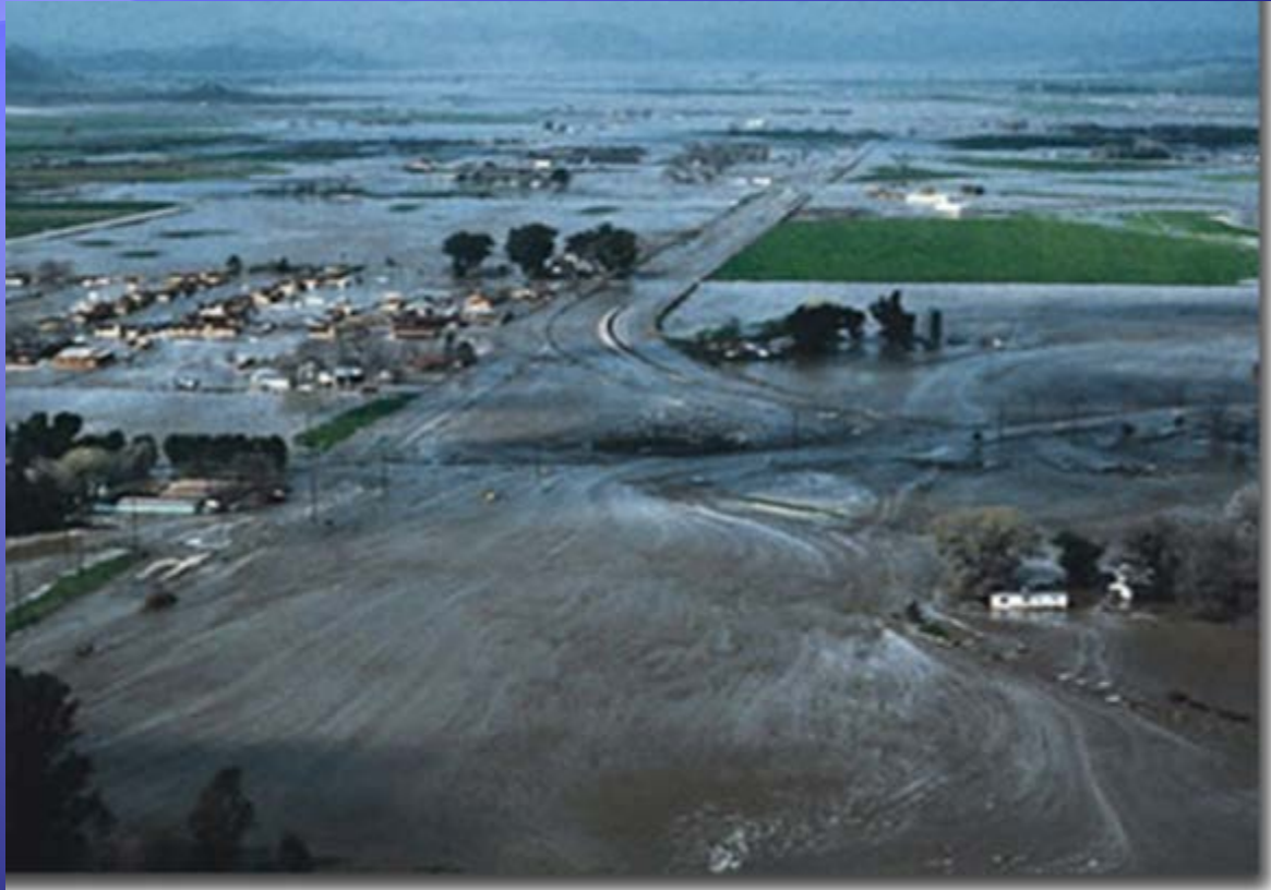
Flooding Due to Breach in Levee on February 21, 1980 Vicinity of State Street and Ramona Expressway
