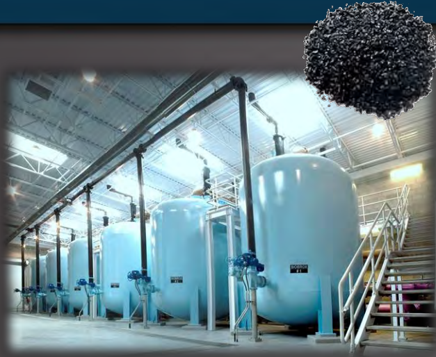
Carbon Adsorption: granular activated carbon (GAC)
