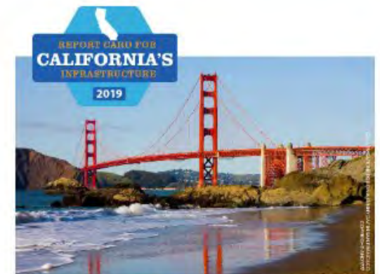
REPORT CARD FOR CALIFORNIA'S INFRASTRUCTURE Region 9 of the American Society of Civil Engineers INFRASTRUCTUREREPORTCARD.ORG/CALIFORNIA
