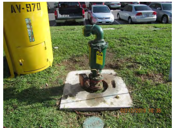
Reach 5 Air Release Valves Map shown (left). A Valmatic VM804 AirVac model shown (above)
