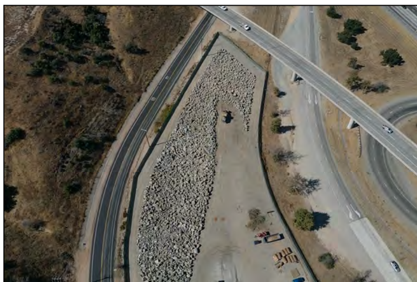
Photo Title: Approximately 7,000 Tons of rock removed are located at Staging Area near intersection of 241/91.
