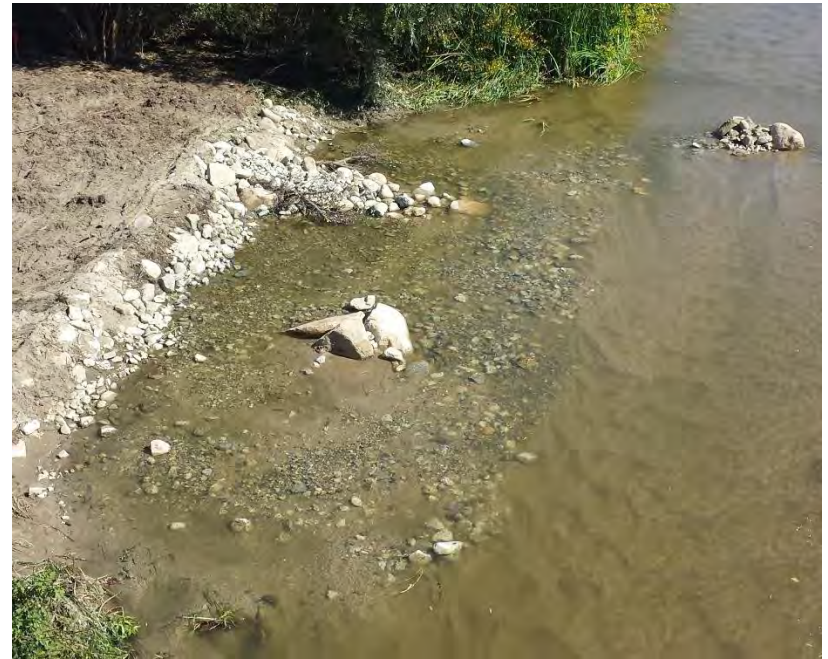
Habitat Structure at Van Buren Boulevard (October 2018)
