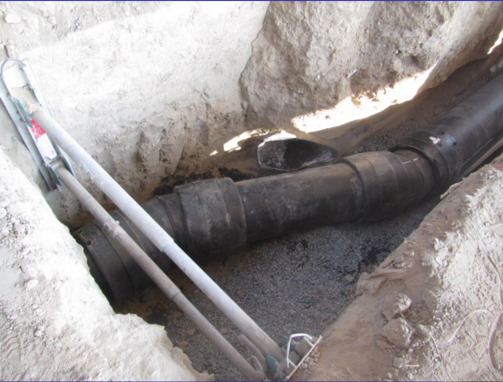
Downstream side connection
