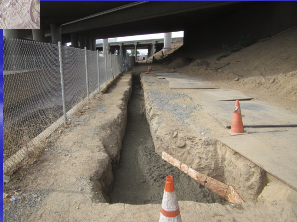
Slurry backfill per Caltrans requirement
