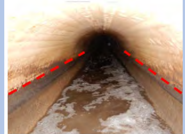
Photo 3-5. Typical water level indicated by slime layer (red dashed line).
