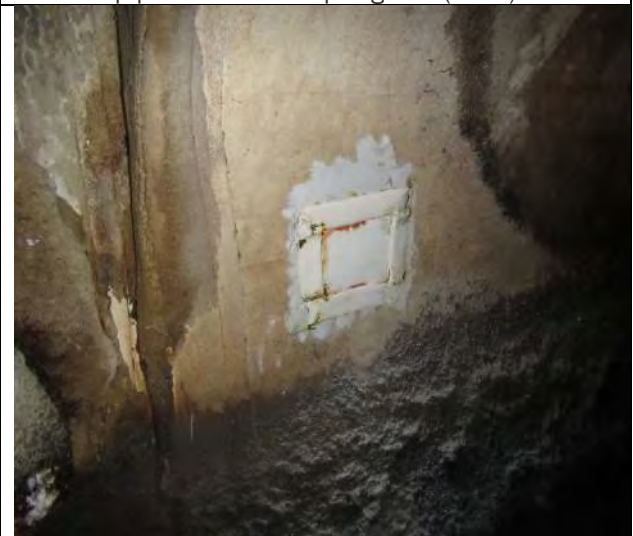
Liner repair at spring line (3:00)
