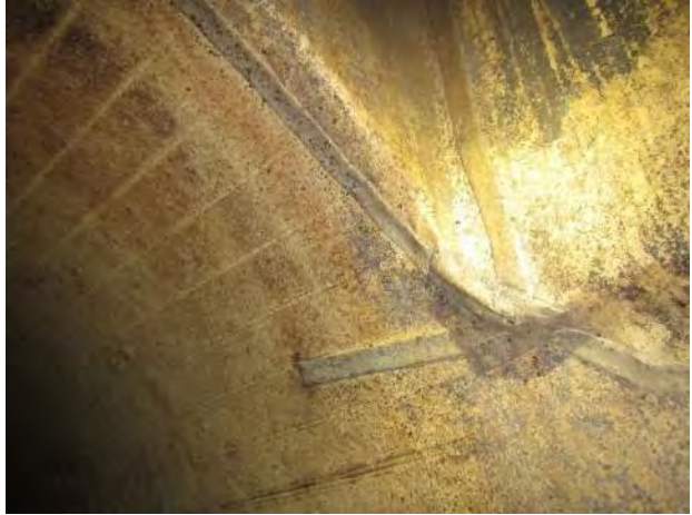
Photo 4-5. Typical main pipe connection in good condition.
