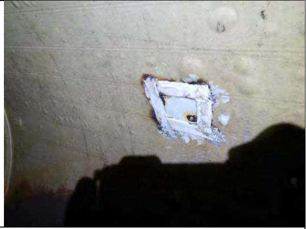
Liner repair at spring line (9:00)
