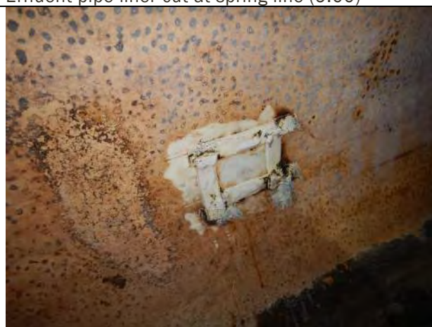
Liner repair at spring line (9:00)
