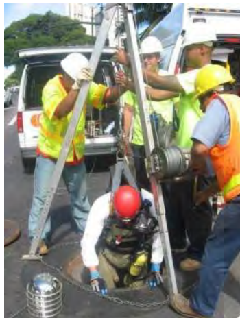
Photo 2-1. Example confined space entry setup
