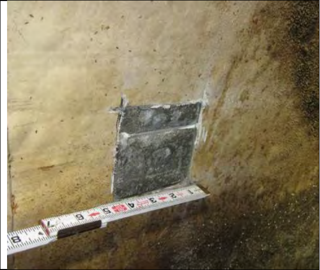
Influent pipe liner cut at spring line (3:00)
