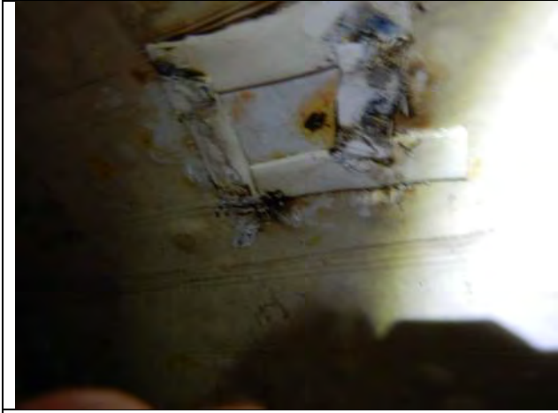
Liner repair at crown (12:00)
