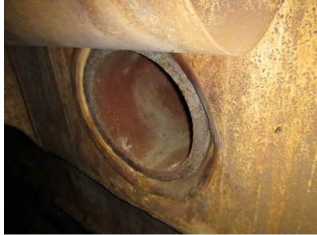
Photo 4-6. Typical lateral penetration in good condition.
