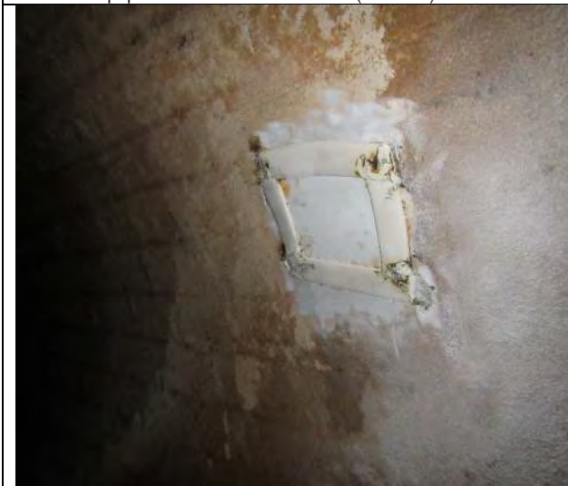
Liner repair at crown (11:00)
