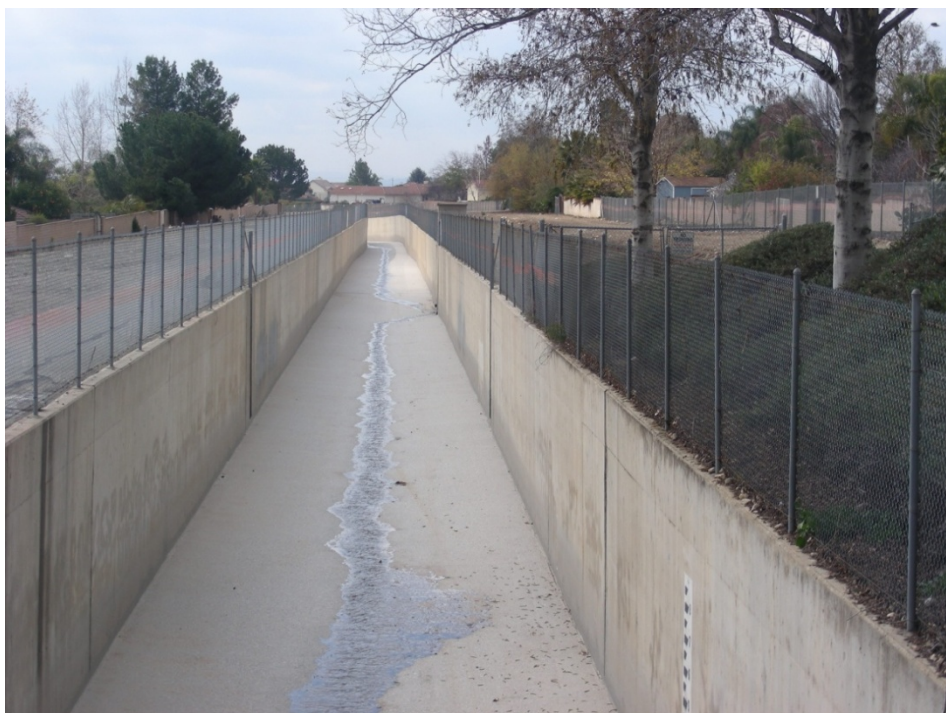
Figure 2 Photo of Demens Channel Survey Location
