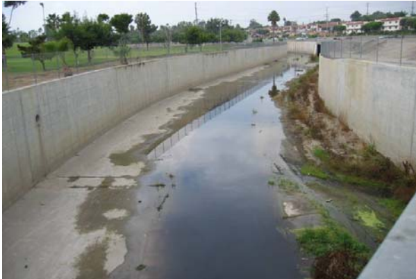
Figure 40 Santa Ana Delhi Channel Downstream from Irvine Avenue
