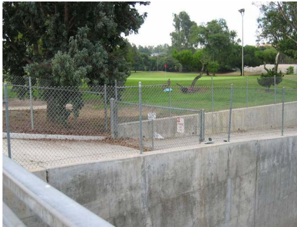
Figure 45 Fencing around Santa Ana Delhi Channel Prevents Access to Waterbody
