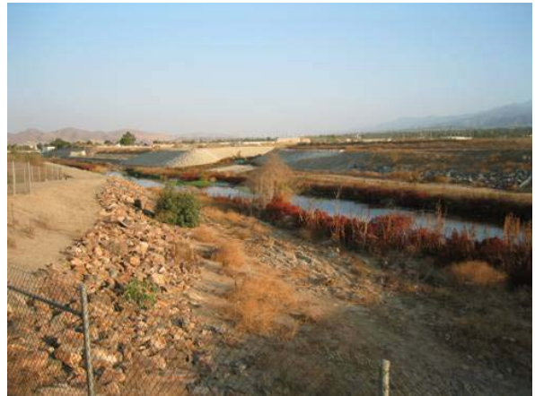
Figure 60 Temescal Creek downstream of Lincoln Avenue bridge, looking upstream
