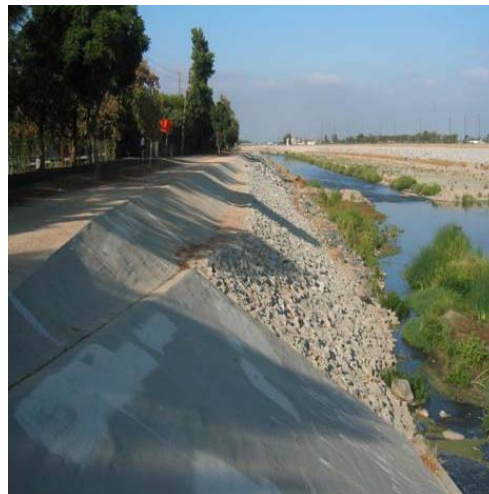
Figure 77 Side Slopes of Santa Ana River downstream of Imperial Highway
