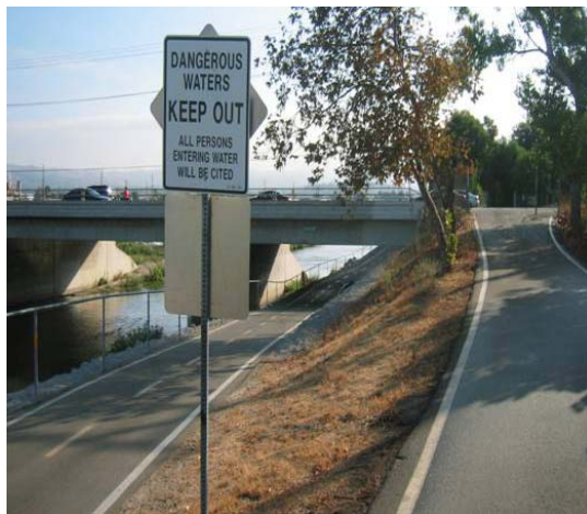
Figure 79 Signs prohibiting entrance into Santa Ana River at the Imperial Highway
