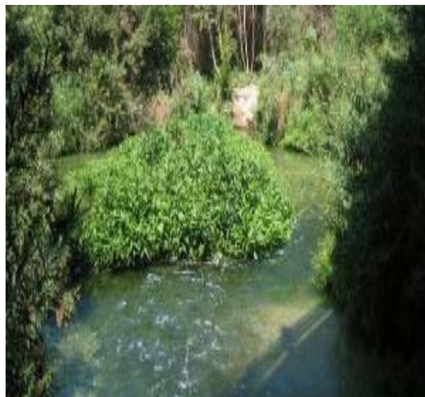
Figure 90 City of Riverside WWTP Effluent Channel
