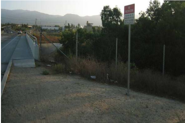
Figure 64 Fencing and signs prohibiting access to Temescal Creek from the Lincoln Avenue Bridge
