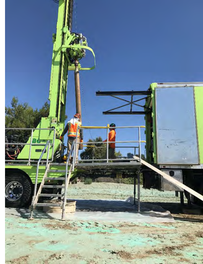
Sonic drilling rig. 8-inch diameter core barrel, telescope down to 200 ft 16
