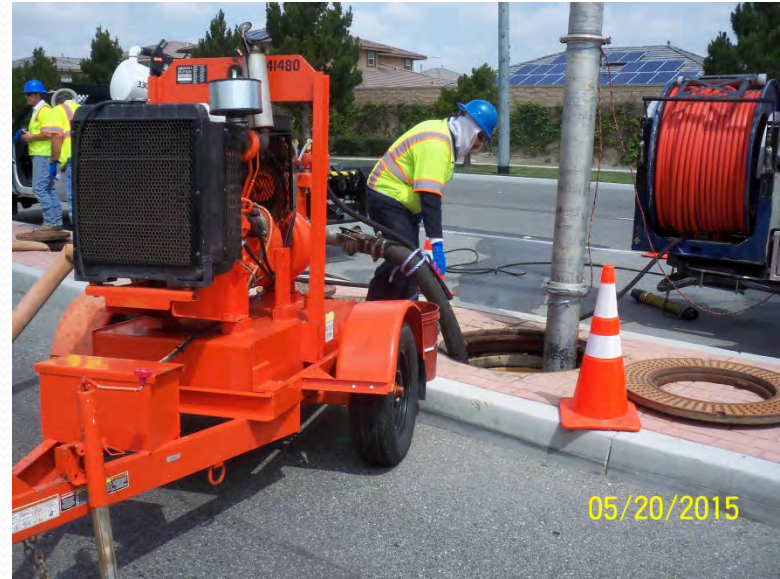
Schleisman Road (Eastvale)
