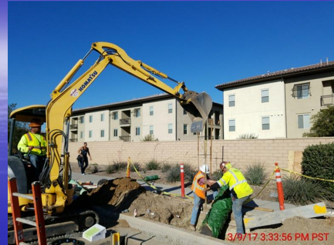
14-inch Lateral Installation
