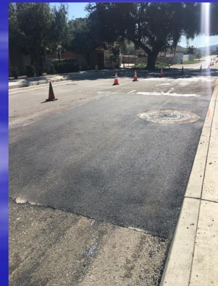
Final Paving Sections 1 - 10
