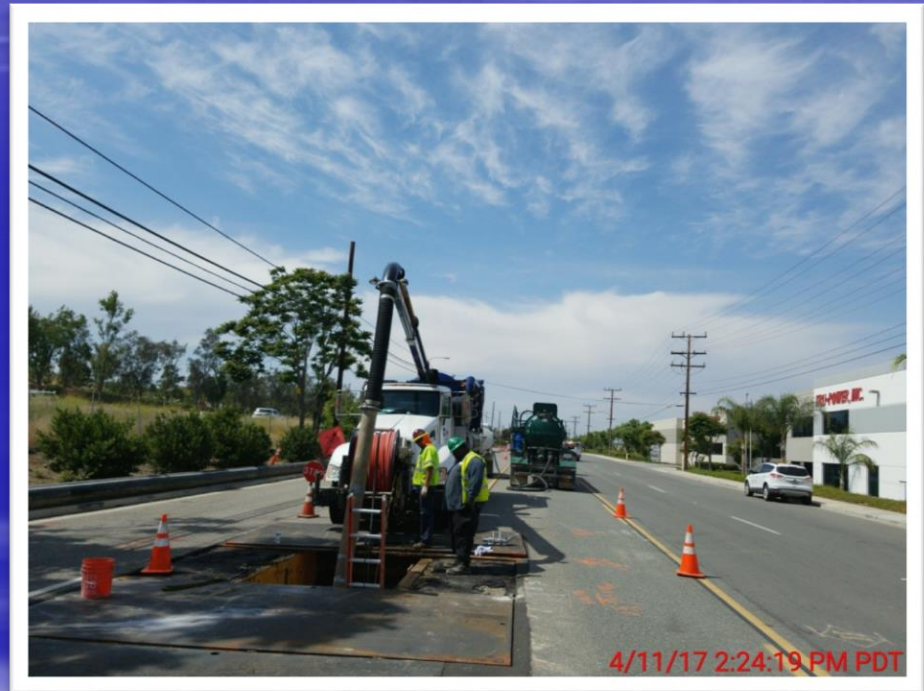
Clean inside Pipe
