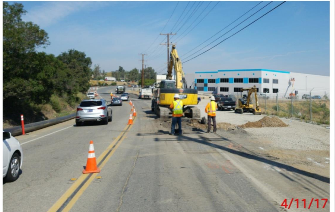
Construct Access Pits
