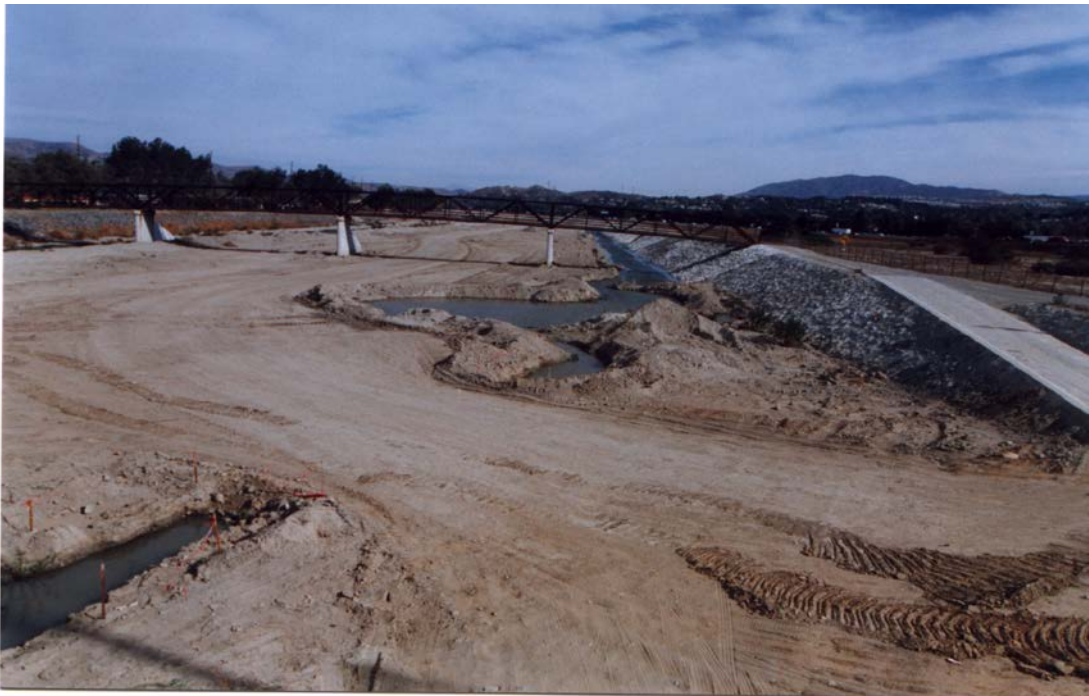
Photo 7. Santa Ana River at Imperial Highway.
