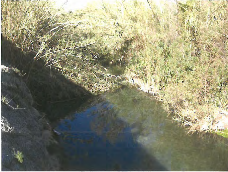
Anza Drain, confluence of drainage and effluent channel.
