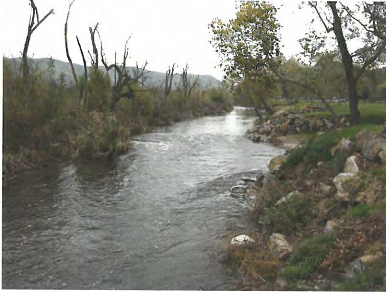
Lower SAR north of Gypsum Bridge, high velocity flows with deep river bottom. Extensive riparian overhangs occur along both banks.
