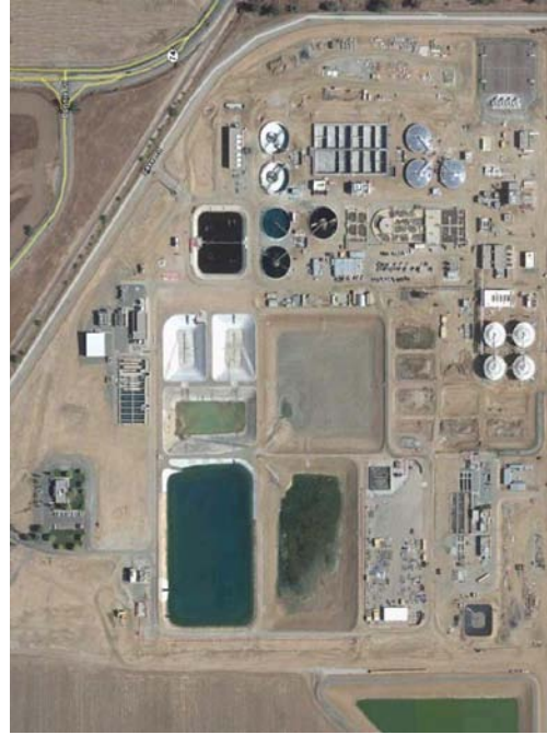
Perris Valley Plant
