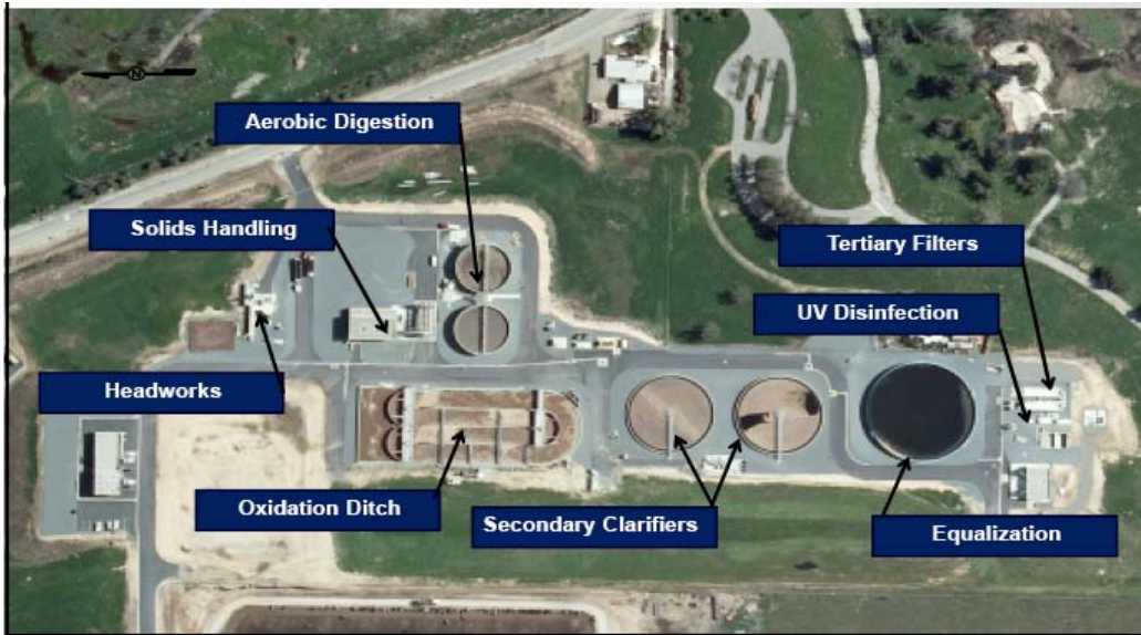
WRCRWA River Road Plant
