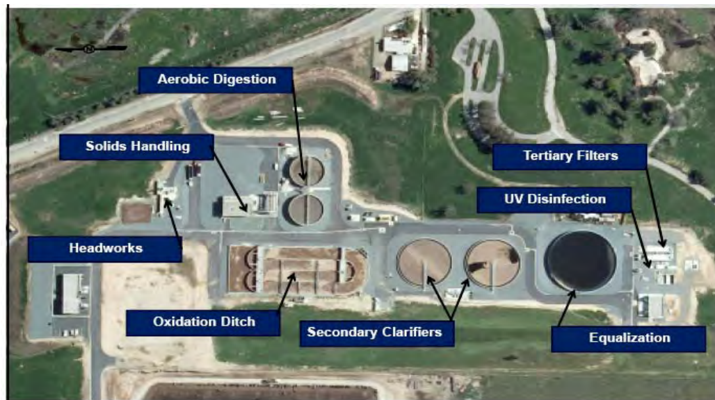
WRCRWA River Road Plant
